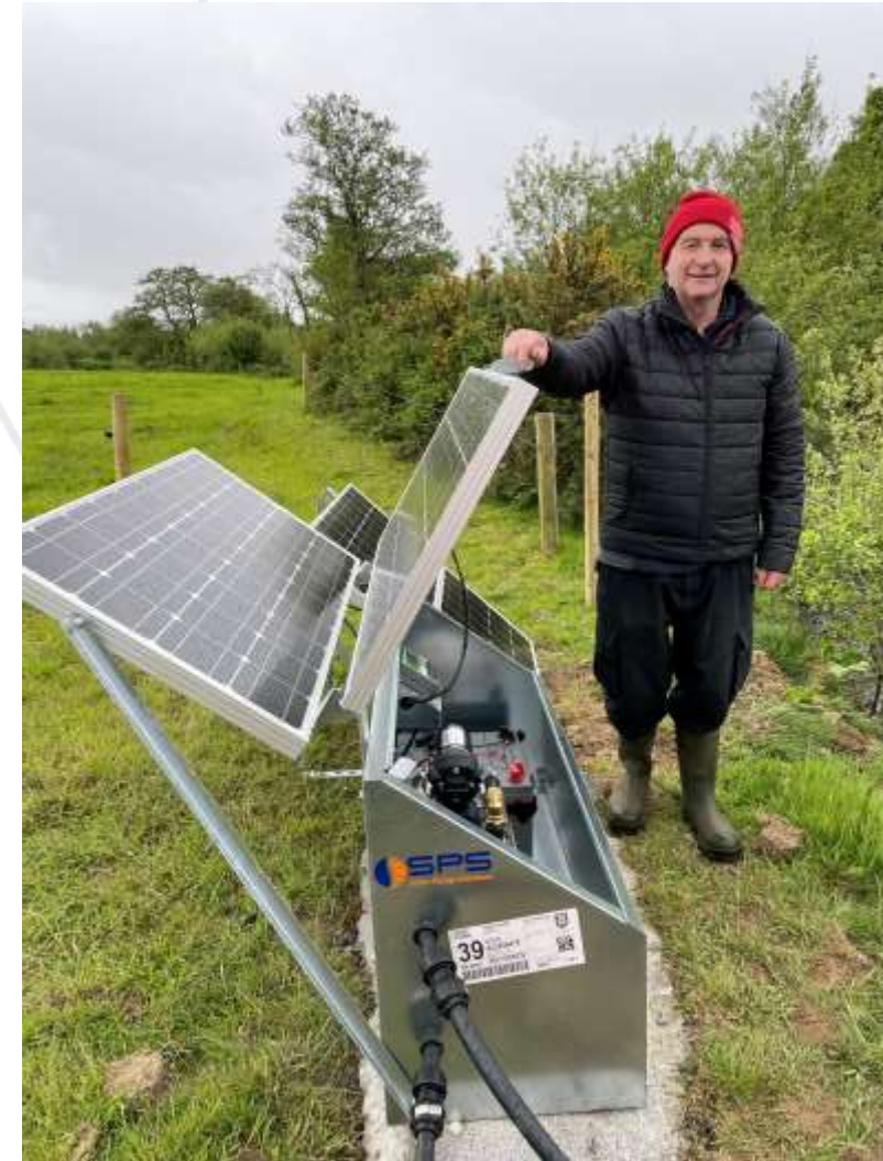
Solar Pump on for alternative drinking point
